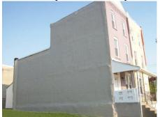
beauty for years to come. The stucco-finished north wall has been cleaned and resurfaced as needed, and coated with two coats of Behr® premium Masonry/Stucco exterior paint in the color Quail Ridge. The front brick
