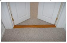
As an added amenity, we install an oak wood threshold at all room door openings so that the carpet will be better maintained at the high traffic areas. Our thought is this: Why have the carpet installer make a glued seam at a doorway, the most highly trafficked area, and thus most likely to tear and fail? If we put in an oak threshold at each doorway, no seaming is necessary, installation may be more easily accomplished, and no seam tears and failures will occur.
