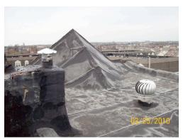
facing wall of the Living Room area. A new torch-down rubber roof has been installed at all roof planes with
